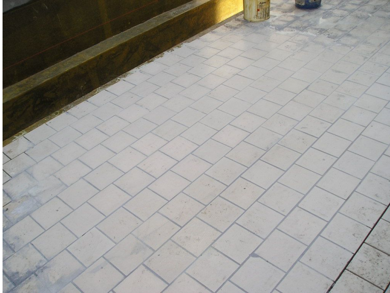
1. Outdoor tiling floor in a chemical plant
